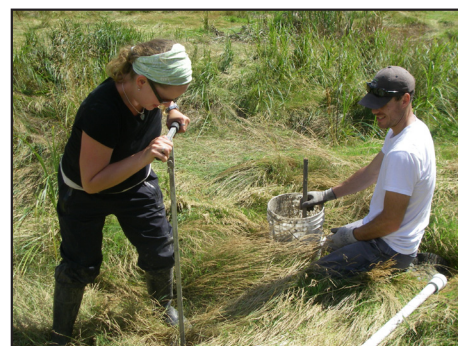
Deep groundwater well installation.
